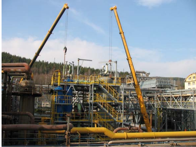
Fig. 8 Process Unit Erection - Heat Recovery from Liquid By-Product Gasification Unit
