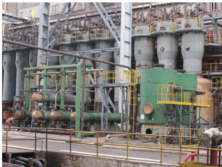
Fig. 1 Heat Recovery Steam Generator Unit for Raw Gas Cooling
