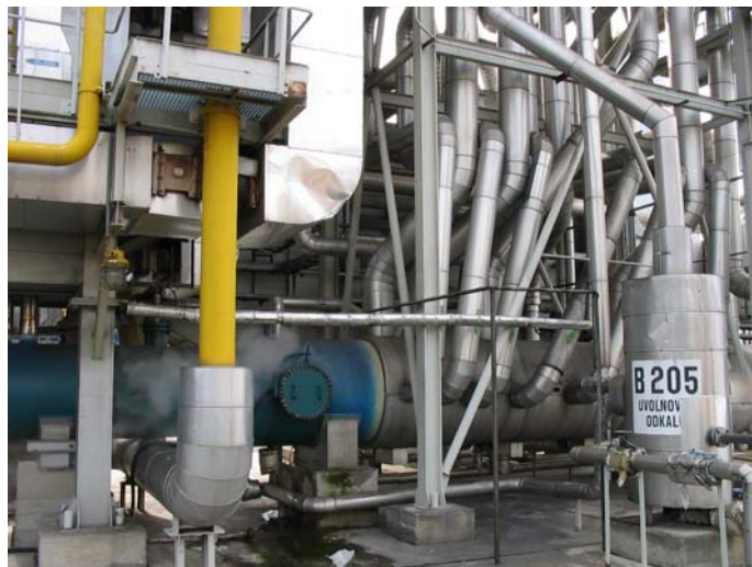
Fig. 5 Waste Heat Boiler in Hydrogen Production Unit
