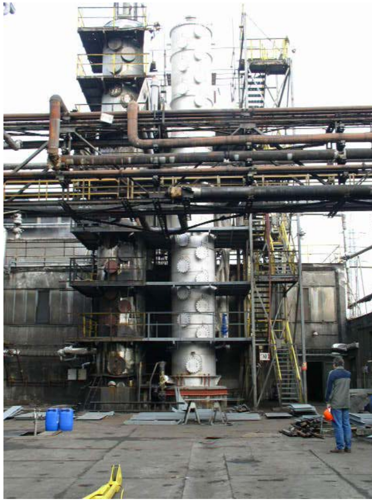
Fig. 9 Erection of Benzole Stripper in Coking Plant Svoboda, Ostrava
