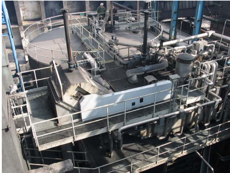
Fig. 3 Tar Sludge Rough Separator, KB9, Coking Plant, Svoboda, Ostrava
