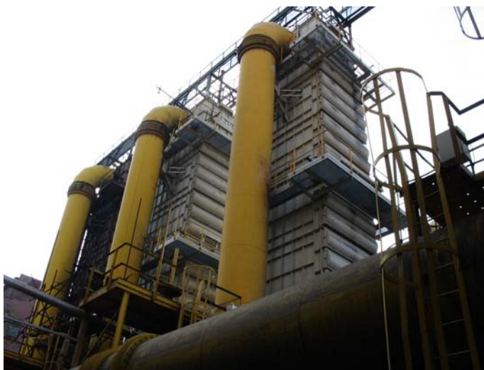
Fig.1 Primary Coolers in Coke-Oven Plant Svoboda, Ostrava
